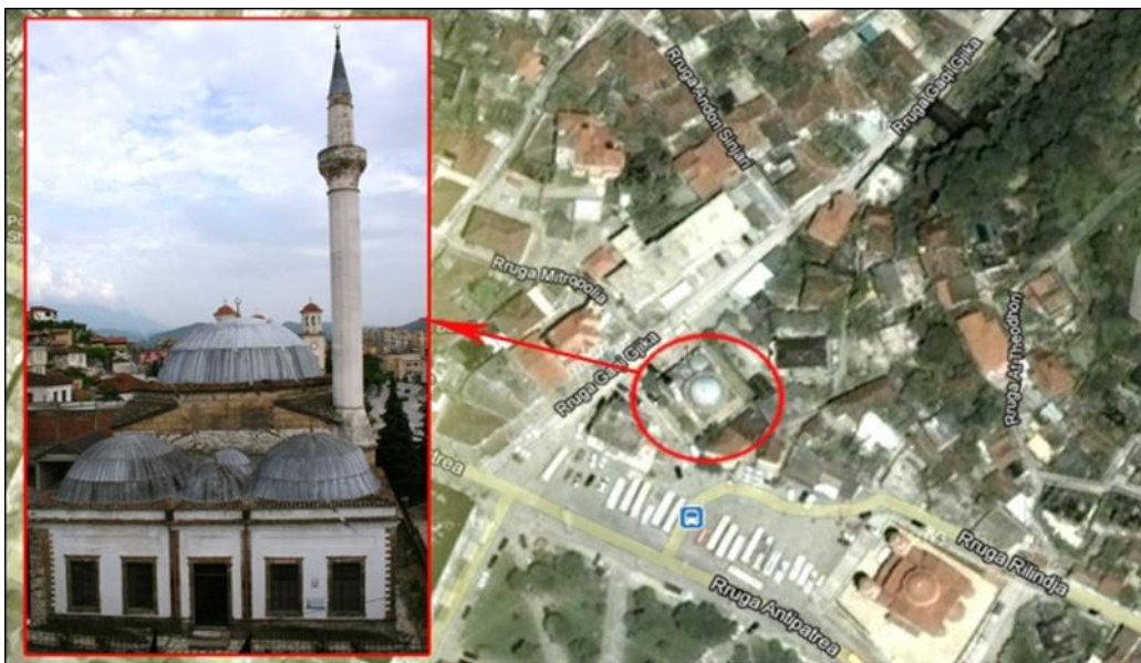
Figure 2. Location and main façade of Leaden Mosque
