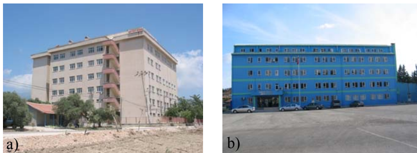
Figure 2. Instrumented buildings (a) The Antakya hospital, (b) The Huseyin Ozbuğday high school
