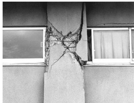
Figure 3. Large window openings and short column
