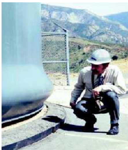
Figure 1. Elephant Foot Buckling
