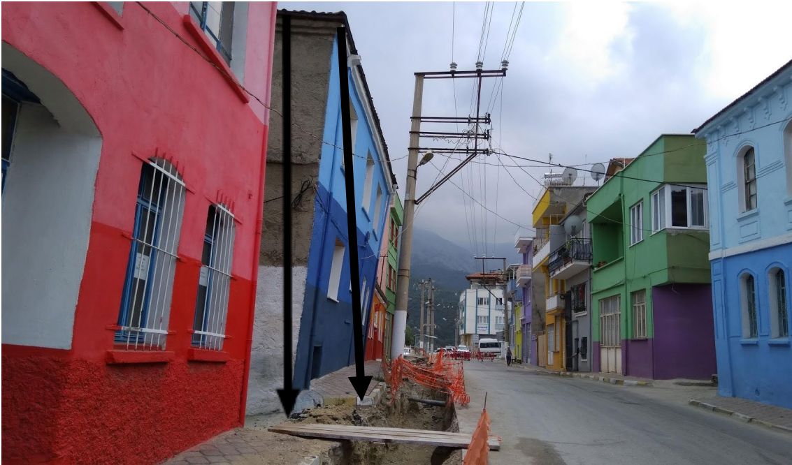
Figure 3. Slide type landslide (a) and landslide induced deformation on dwellings in Babadağ (b).
