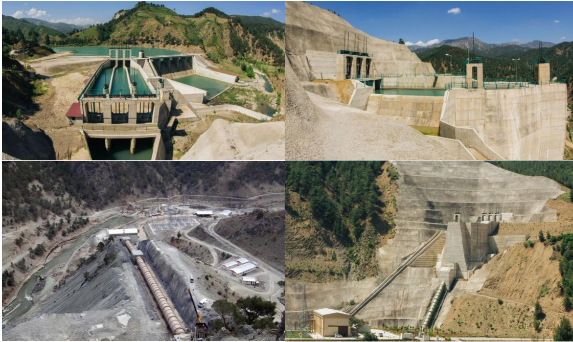
Figure 1. View Of The Run-Of-River Hydroelectric Power Plant From Different Angles
